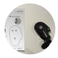
Remove template and drill pilot holes (ideally 1/16" diameter).
